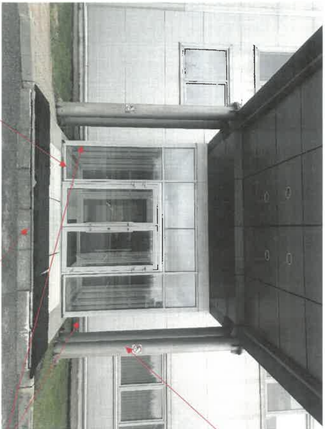
* Drain channel Installation On both sides
